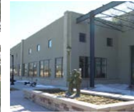
Copper Pointe , 10500 Copper Ave. NE, was built in 1971 as a telecommunications equipment plant then closed in 1993. Vacant until 2008 when it reopened following a major renovation, it now houses Copper Pointe Church and Brown Mackie College as two of its major tenants.
